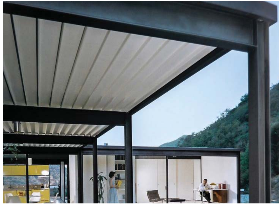
BLACK METAL STRUCTURE
